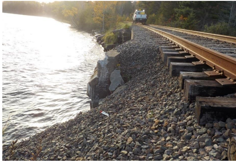
Figure 5: Typical erosion and undermining of track support at mile 46.9 Sydney.
