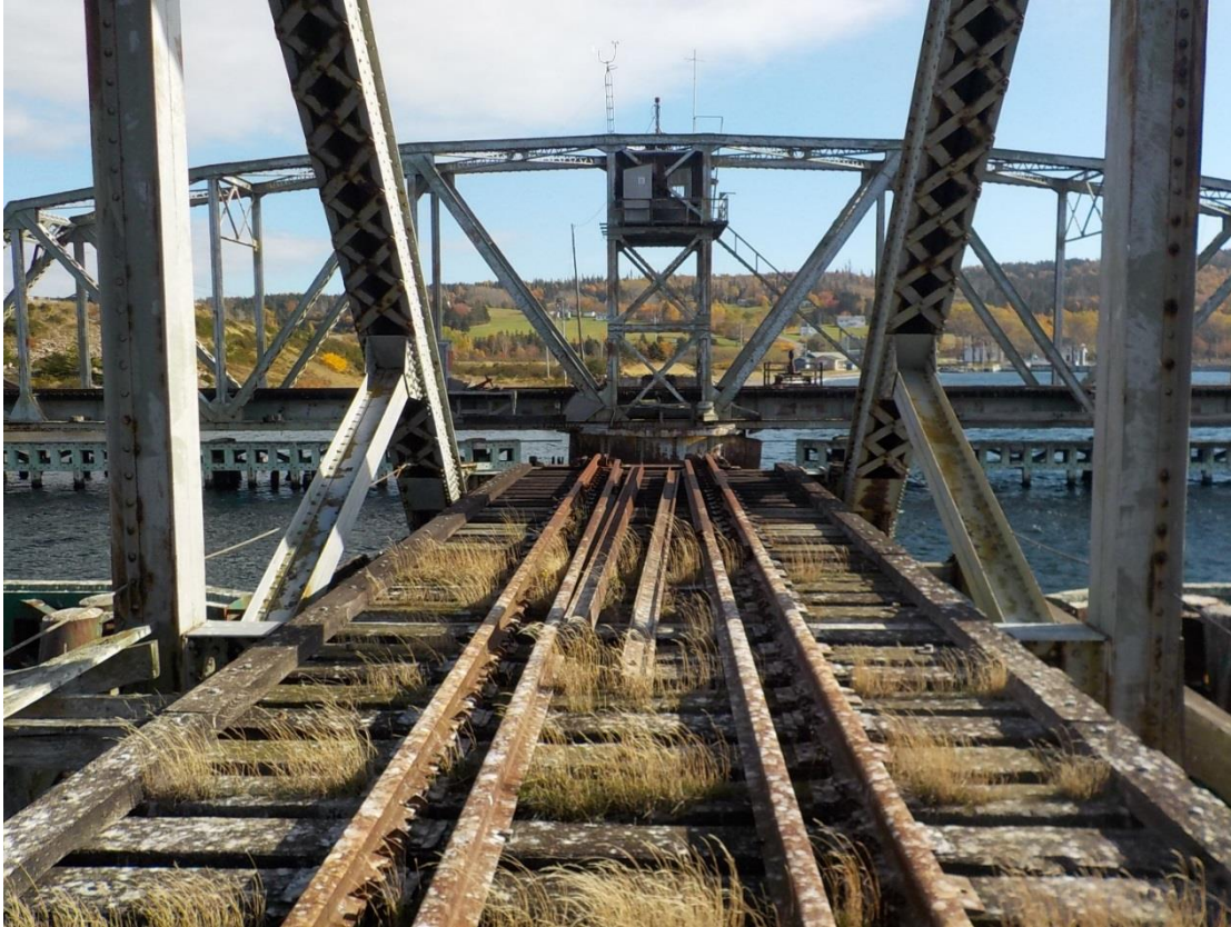
Figure 6: Rotten and split ties with significant vegetation at 57.8 Sydney.
