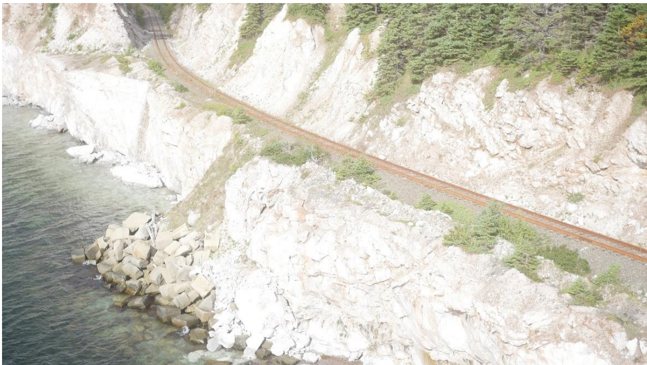
Figure 4: Erosion of gypsum cliff supporting track, approx. mile 53.
