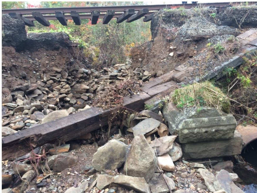
Figure 3: Wash-out and destroyed culvert at mile 110.1.
